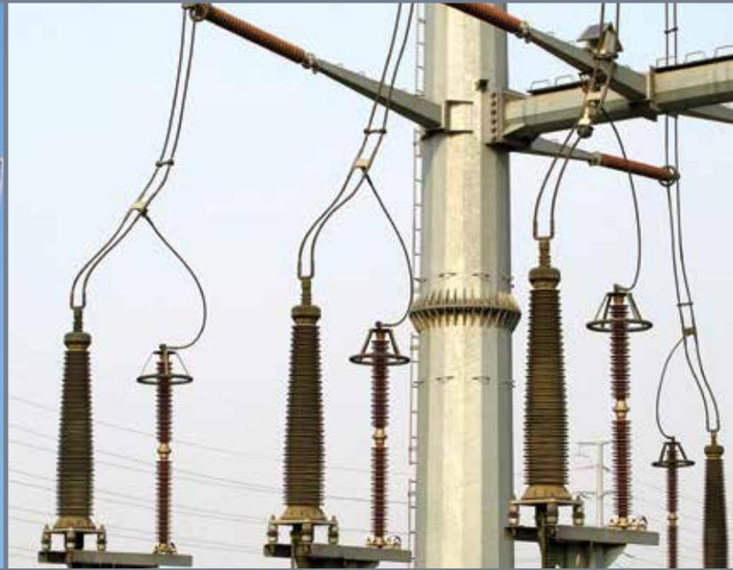
The traditional design of most outdoor cable terminations at the higher voltages has been based on a hollow core insulator made from either porcelain or a composite tube covered by silicone sheds. The insulators in both cases are equipped with a field control element made from silicone rubber and are filled with an insulating liquid or gas.
