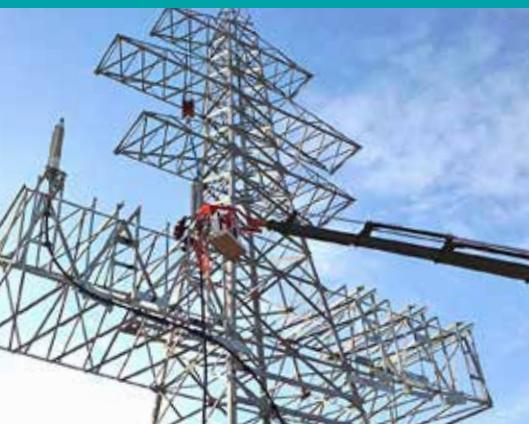
Lifting 170 kV dry type outdoor termination with no need for scaffold on tower.
